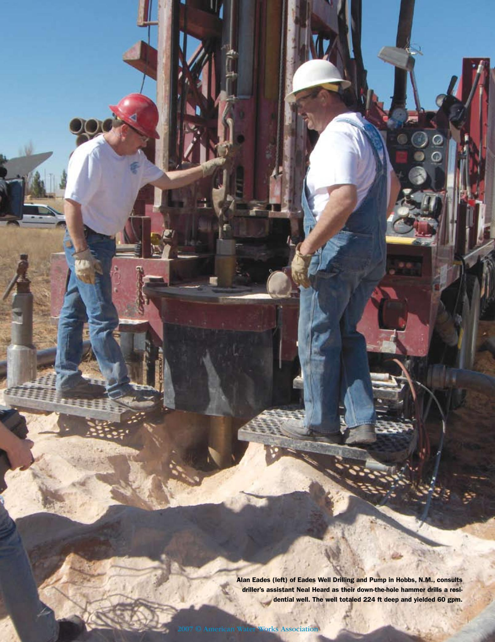
Alan Eades (left) of Eades Well Drilling and Pump in Hobbs, N.M., consults driller's assistant Neal Heard as their down-the-hole hammer drills a residential well. The well totaled 224 ft deep and yielded 60 gpm.
